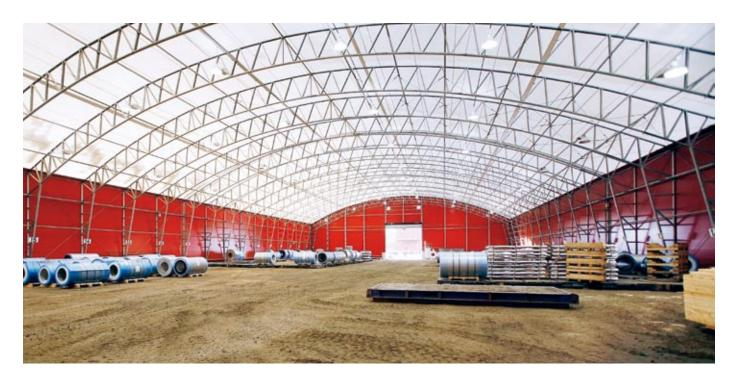
for 20 years. De Boer Scandinavia delivered a specially designed solution involving two halls - one 40 × 80 m and one  $30 \times 30 \,\text{m}$  – linked by a small corridor that acted as a secure barrier. On one side was a large, dry storage room and on the other a loading area with two sides kept
